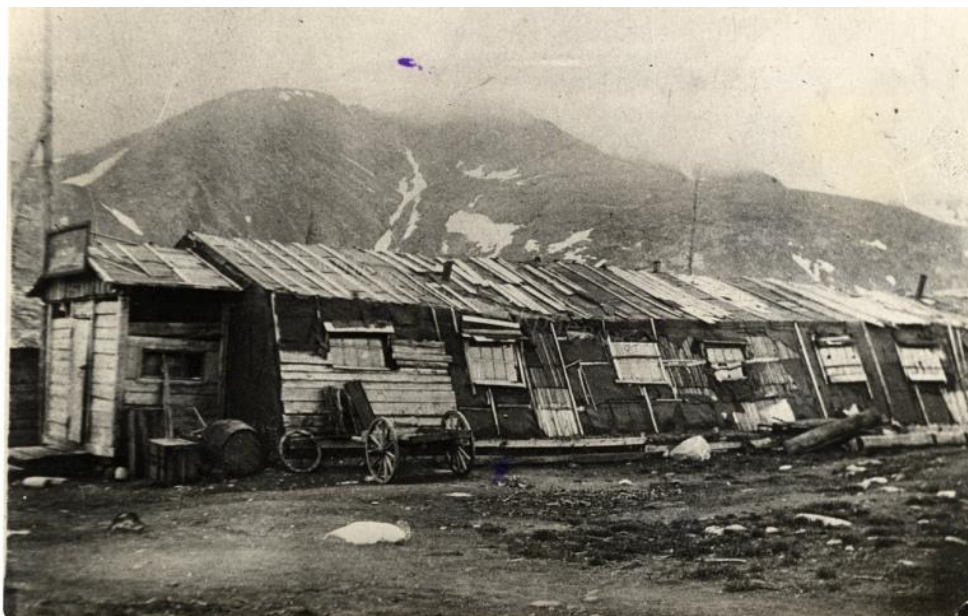
Fig. 1. Shalmans , the first dwellings in Khibinogorsk (structures made of boards upholstered with tar paper), early 1930s. Source: collection of The Local History Museum of Kirovsk
